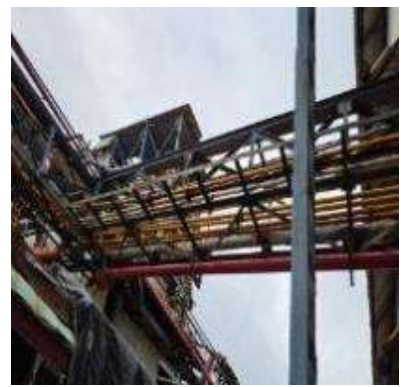
Pipeline found in rusty condition needs to be painted
