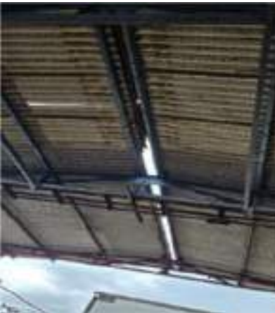
Asbestos sheet of roof found leaking, needs to be repaired. Also, support structure to be painted
