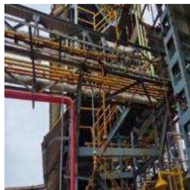
Pipeline found in rusty condition needs to be painted
