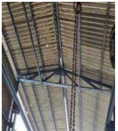
Asbestos sheet of roof found leaking, needs to be repaired. Also, support structure to be painted
