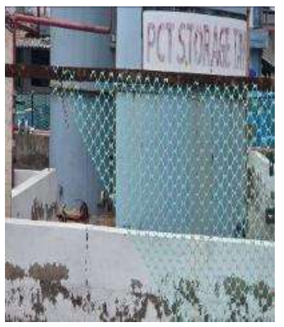
PESO license area needs to be maintained as per the license conditions, like display of license number with validity, adequate size fencing, entry for authorize persons, warning signages
