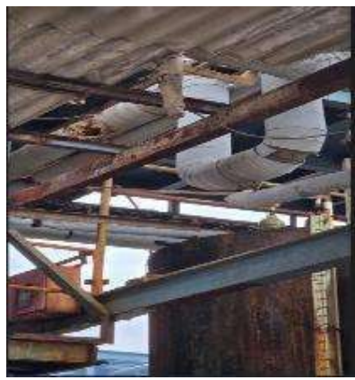
Insulation found damaged needs to be repaired & structure rusty needs to be painted
