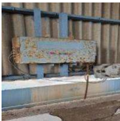
Panel rusty needs to be repaired
