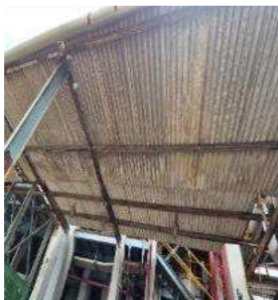
Insulation found damaged needs to be repaired & structure rusty needs to be painted
