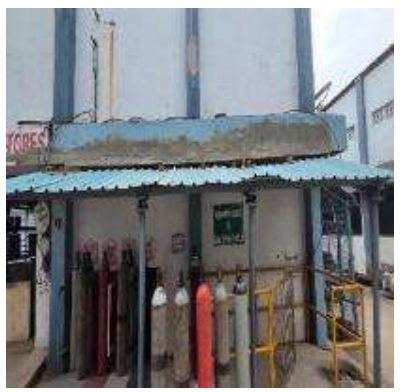
Cylinders to be kept safely away from sunlight as per GCR rules.
