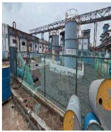
PESO license area needs to be maintained as per the license conditions, like display of license number with validity, adequate size fencing, entry for authorize persons, warning signages
