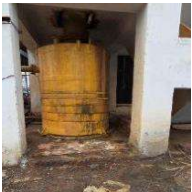
Chemical spillages to be cleaned, also housekeeping needs to be maintained
